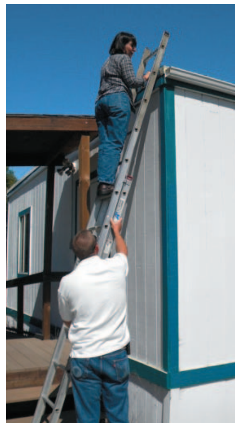
Harry Bunfill assists Robin Kulakow as she inspects the new roof installed by HB Urethane Roofing.
